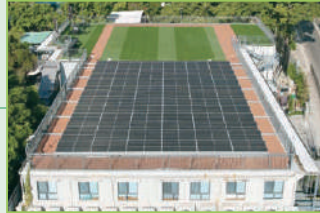
Solar panel installation for more renewable electricity generation is under planning
