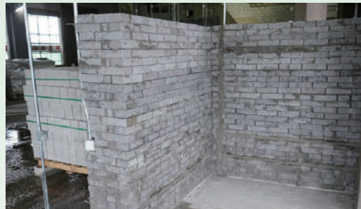
Wall made of the carbon fixation bricks (taken at O-PARK2 site)
